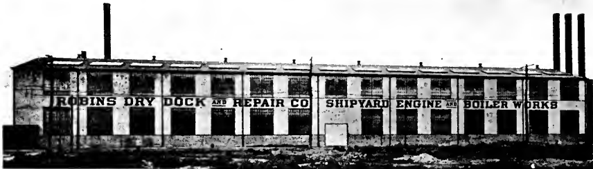
New machine shop recently added to the Robins plant.
